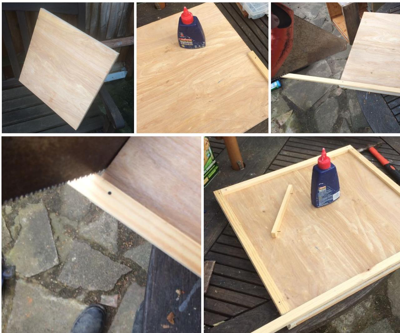
*Making a crownboard. From the top left: a plain 46cm plywood board; temporarily nailing the strip of to one edge in the corner; trimming the strip so it's flush with the edge; repeat for side 2; repeat for side 3; remove the temporary strip and complete slide 4.*
