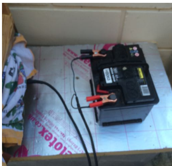
Connecting the battery.
