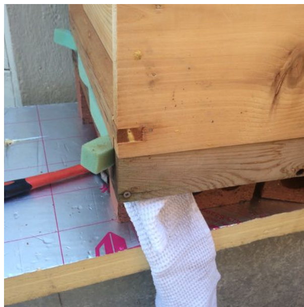
Extra sealing needed on wooden floors.
