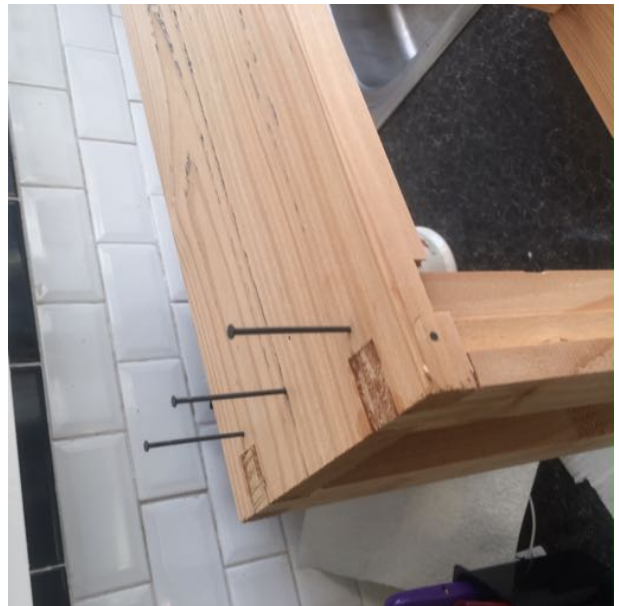
Even more nailing.
