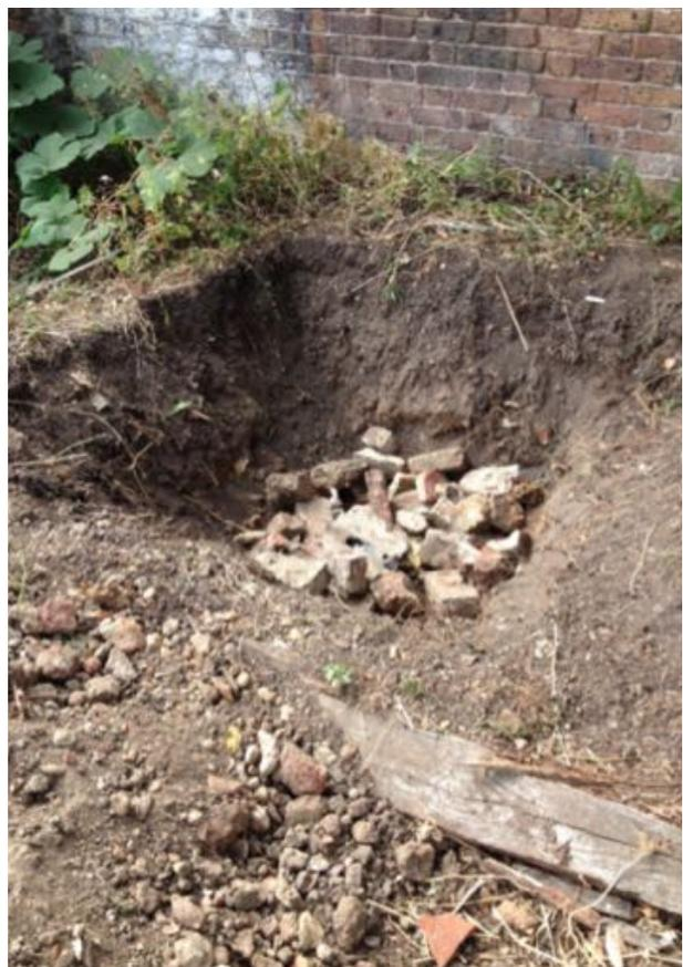
*We put bricks at the bottom of the pit to create a sump to collect the honey from the frames (burning honey is evil).*
